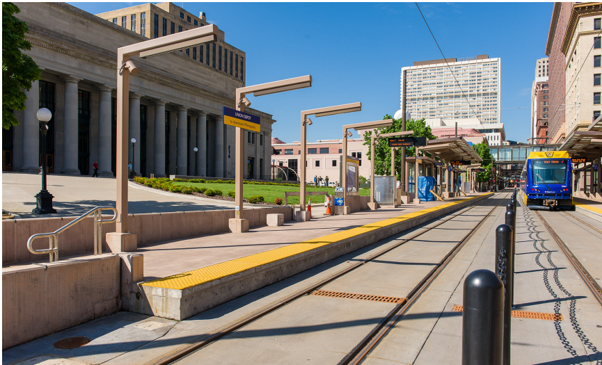
The recently renovated Union Depot in St. Paul is a hub for Amtrak, light rail and bus transit.
